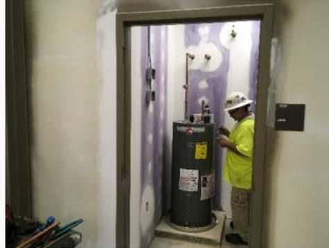
Installation of Water Heater
